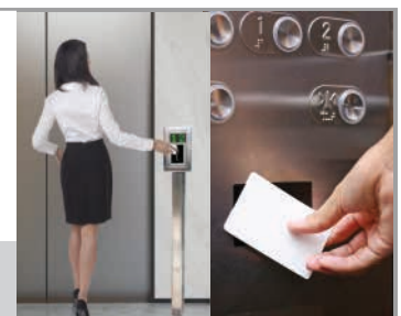
Card reader in Destination Operator Panel and Car Operator Panel
